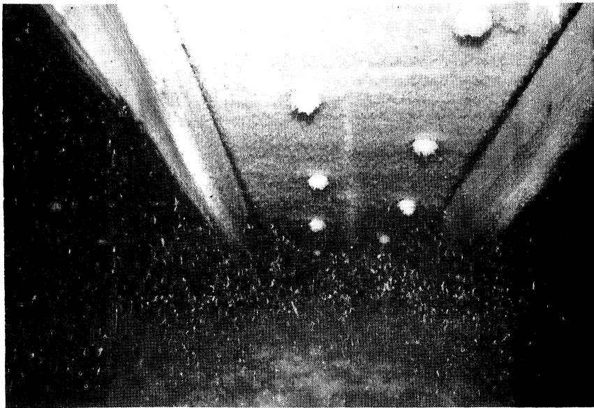
Fig. 1 Illustration of frost build-up on the underside of roof sheathing. (This photograph was provided by Vince Meyer of Diversified Insulation.)
