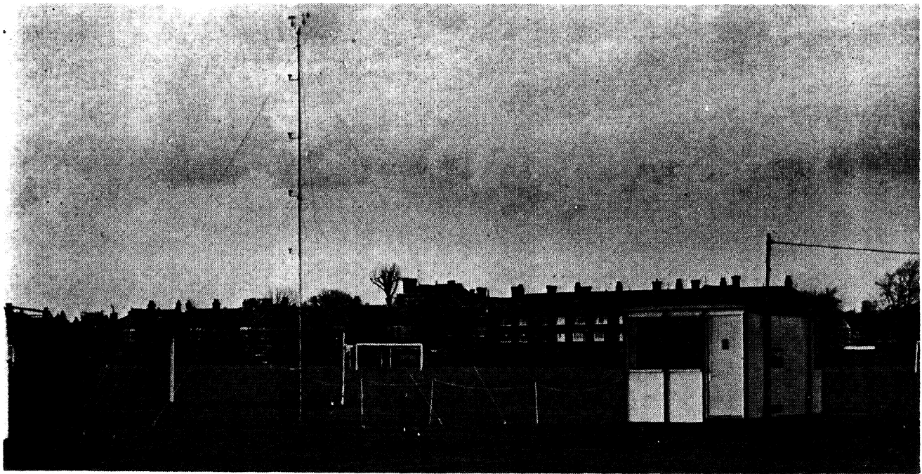
Fig 3: Portakabin structure on site (showing mast for measuring wind profile and turbulent intensity).
