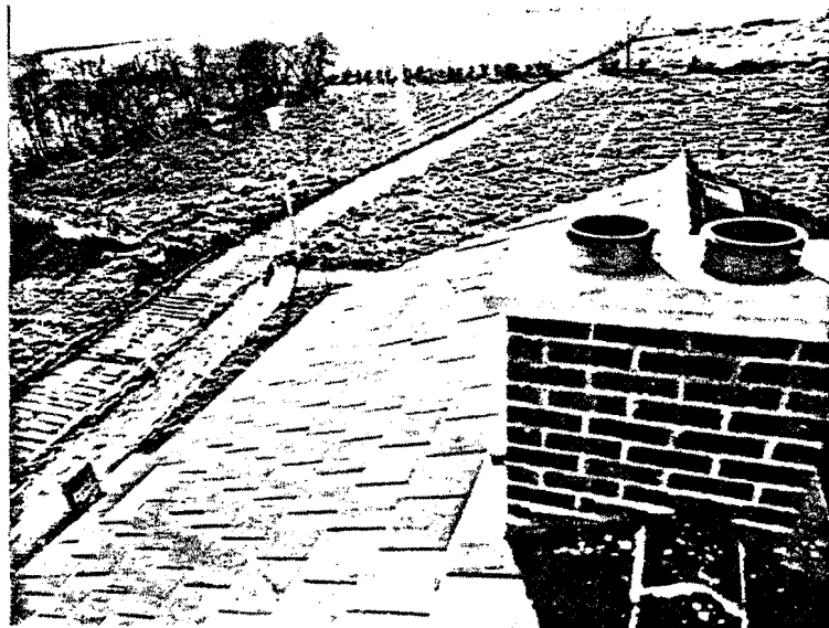
Fig.12. Transducers mounted on the roof of house 70.
