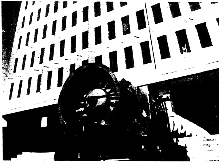
Fig. 1 Air supply fan and ductwork outside test building
