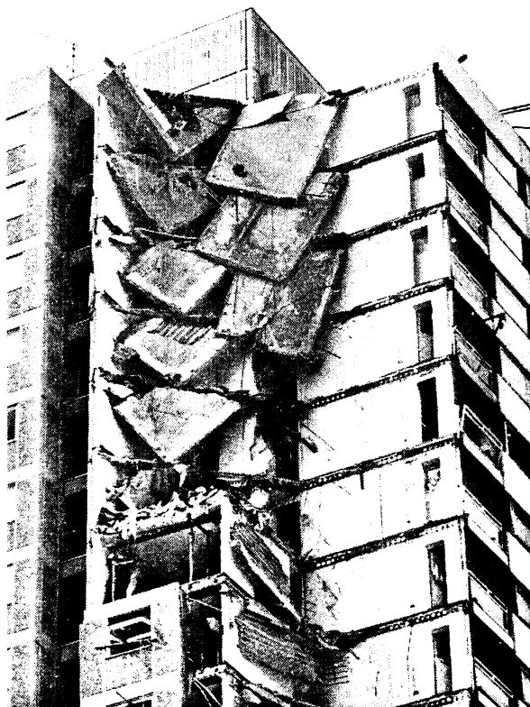
Fig. 4. Damage at Ronan Point.
