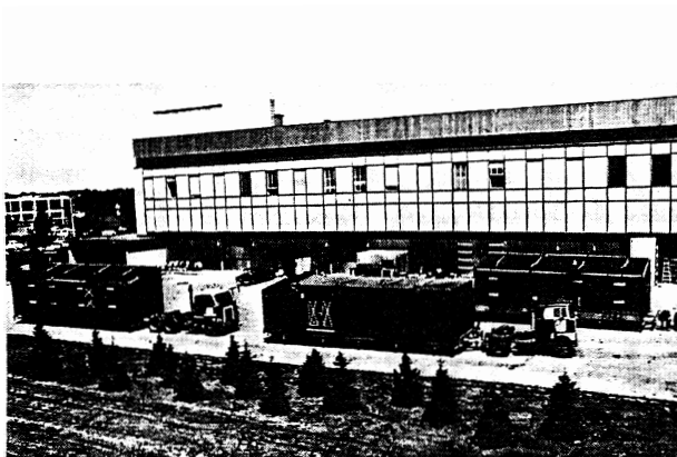
FIGURE 9. Arrival of three modular units at NBS.
