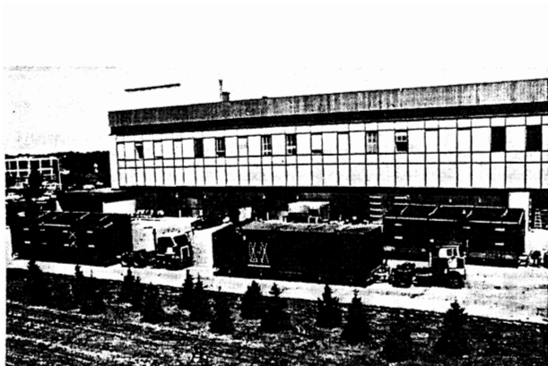
FIGURE 9. Arrival of three modular units at NBS.
