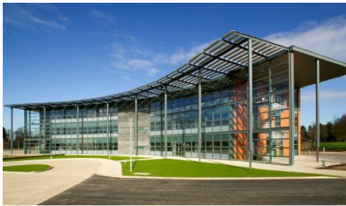
Figure 5: Red Kite House office building
