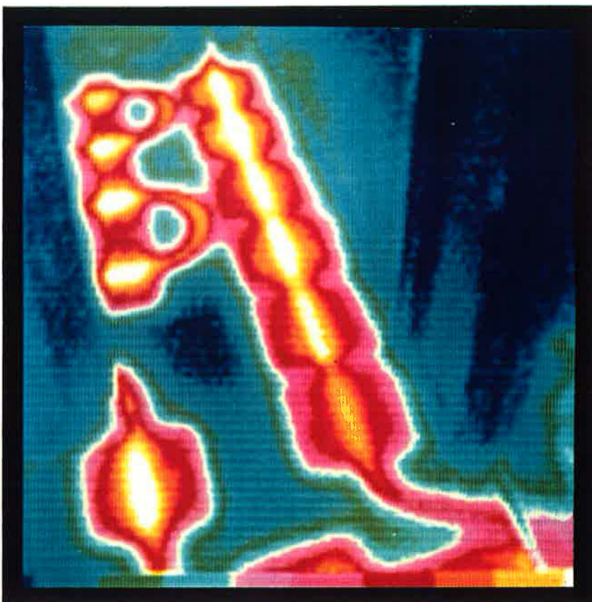
Figure 29(b) As Figure 29(a) but first floor installation showing heat spreader plates
