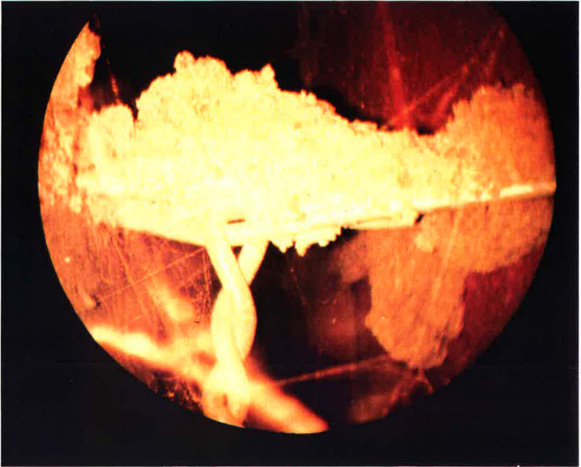
Figure 37 Optical probe photograph showing a mortar 'bridge' resting on a wall tie
