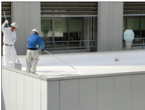
Coating the high reflectance paint on the roof of objective building
