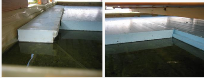
Winter mode: the water is removed and replaced by insulating panels.
