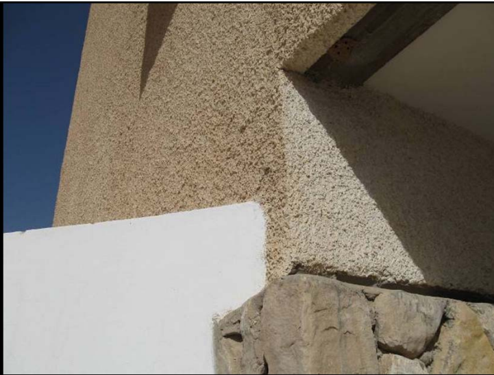
Detail of building at Kibbutz Yotvata: The flat concrete surface at bottom left was recently painted white. The textured plaster in the hallway is still light in color whereas exterior plaster exposed to dust has darkened.
