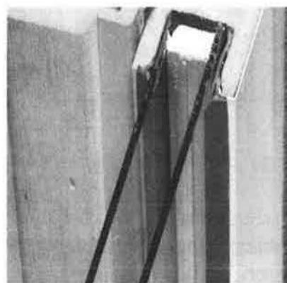
Figure 7-26 — Hollow aluminum edge spacer filled with desiccant.
